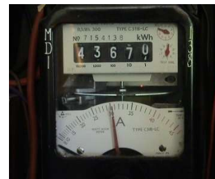
Induction disk meter with Maximum Demand (dial at bottom)
